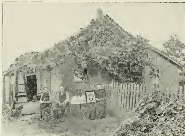
AN EARLY DAY DWELLING IN RICHLAND COUNTY Built of clay and straw mixed
